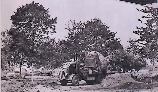
Ropes, pulleys and motors make planting 30-ton red maple in Flushing Meadow Park a simple matter
