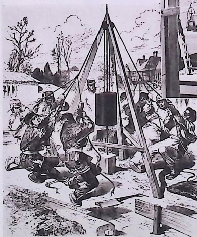
At Philadelphia Centennial of 1876 Japanese workmen drove home foundations for their building with elbow grease
